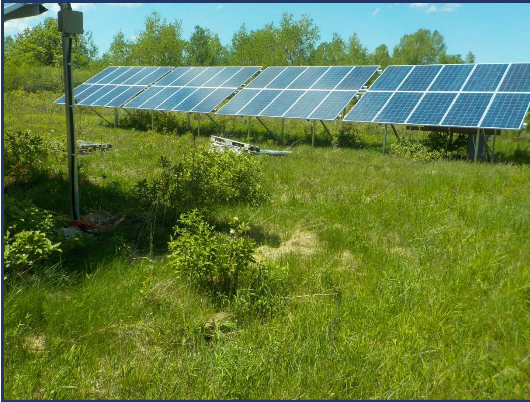
Photo 5: Area Assessed by Test Pit Survey at 5m Intervals, Facing West
