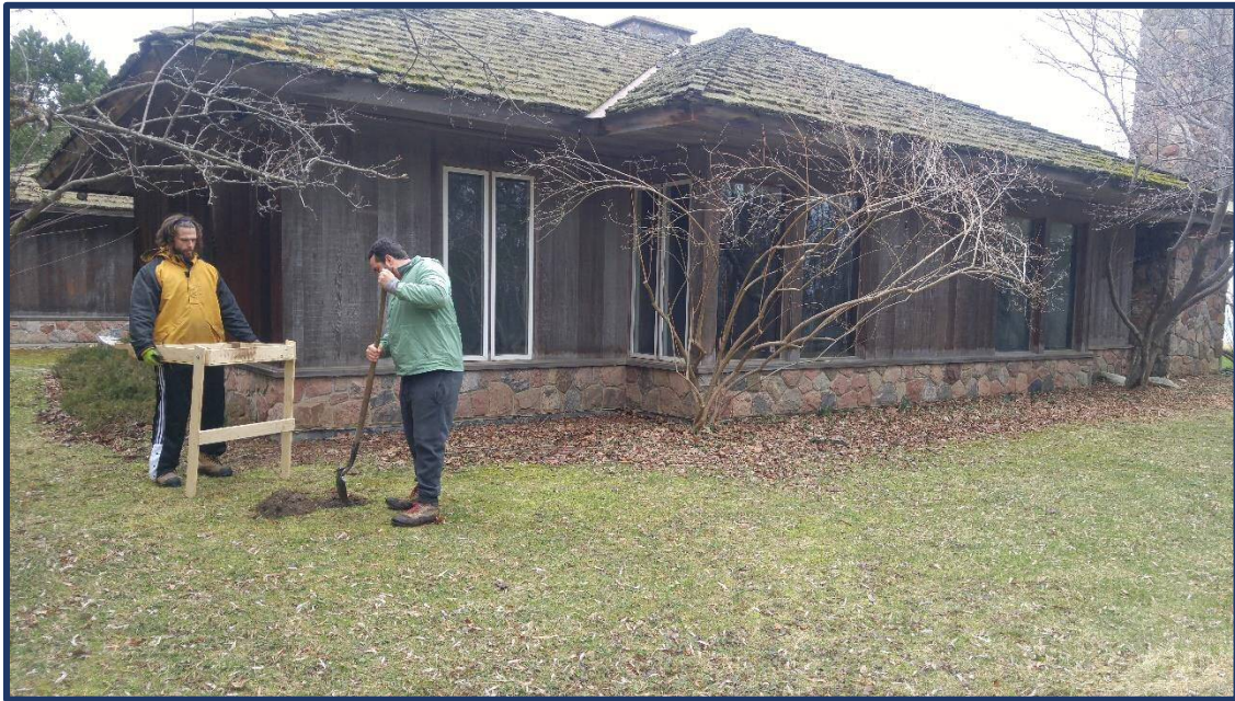
Photo 13: Test Pitting Around Structure, Facing East
