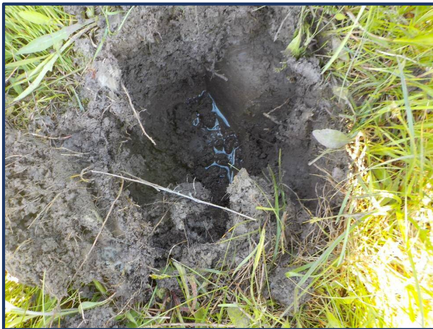
Photo 16: Example of Test Pit West end of Property, Facing South
