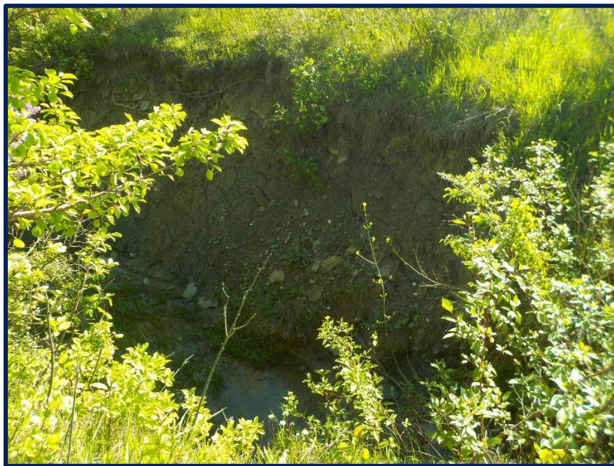
Photo 20: Water Running Through Property, Facing East
