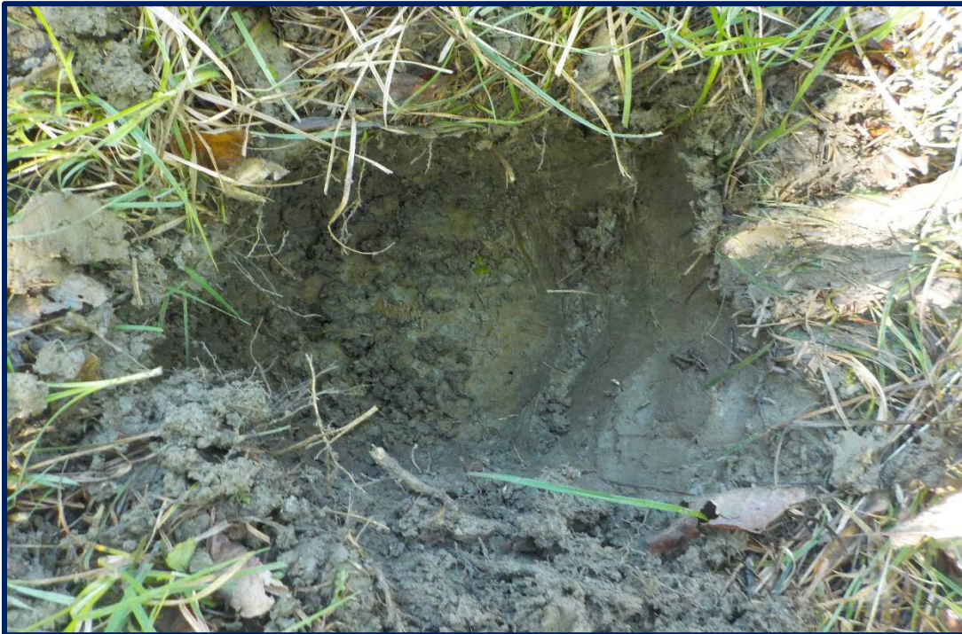
Photo 14: Typical Test Pit Around Structure, Facing West
