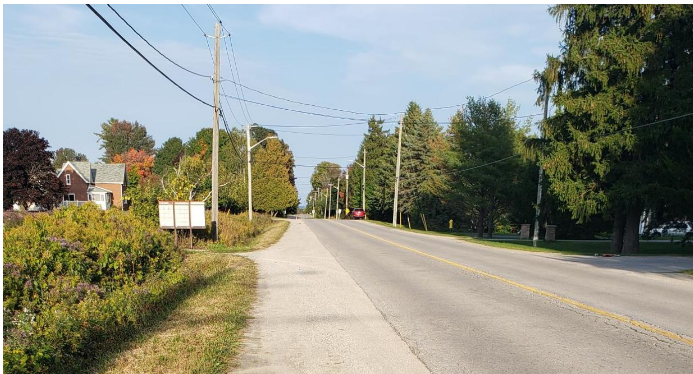
Looking east along Miller Street from the site access
