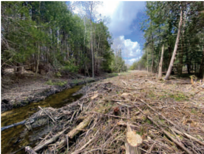
Clearing Working Space and Removing Obstructions
