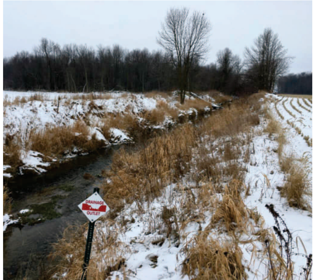
Example of an open Municipal Drainage System
