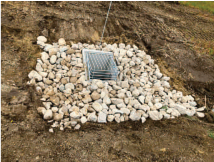
Ditch Inlet Catch Basin
