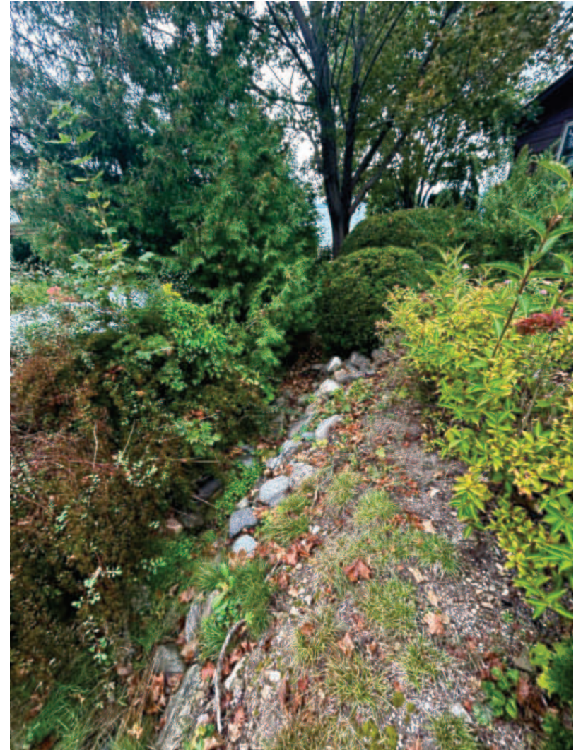
Flow Route on the Deskur / Campbell Property Line September 2024
