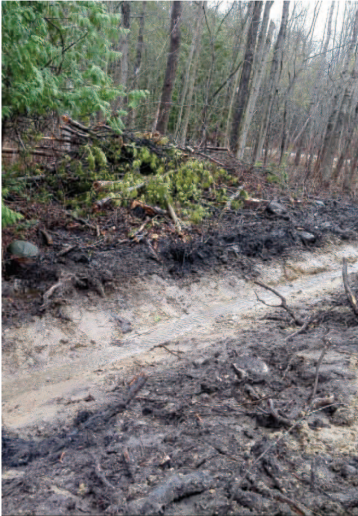
Artley Road Ditch Cleanout April 2022
