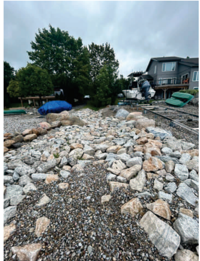
Erosion Protection on the Deskur / Campbell Property Line September 2024
