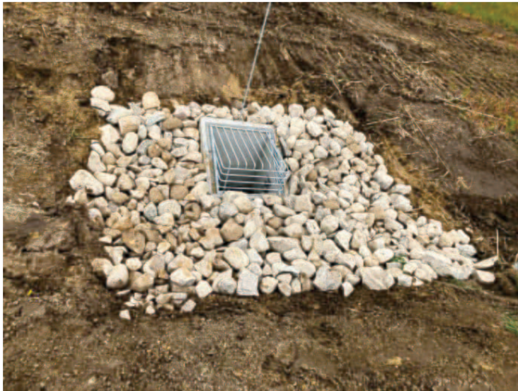
Ditch Inlet Catch Basin
