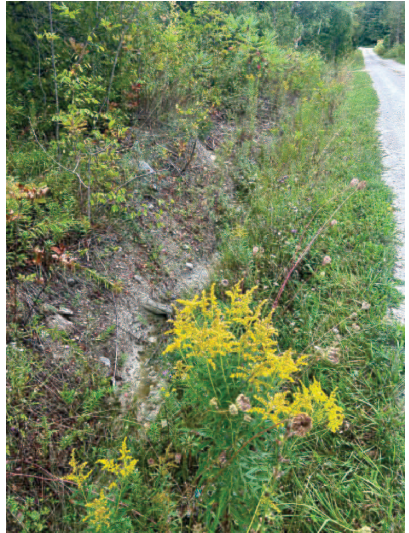
Artley Road Ditch September 2024
