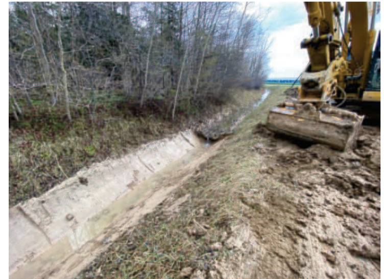
Channel Deepening and Spoil Leveling
