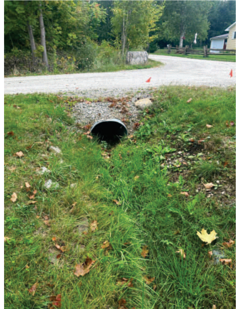
Culvert Under Paradise Bay Road September 2024
