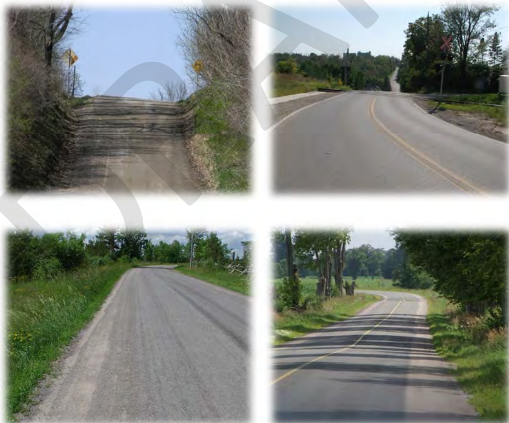
Figure 3.2: Potentially Substandard Vertical and Horizontal Alignment
