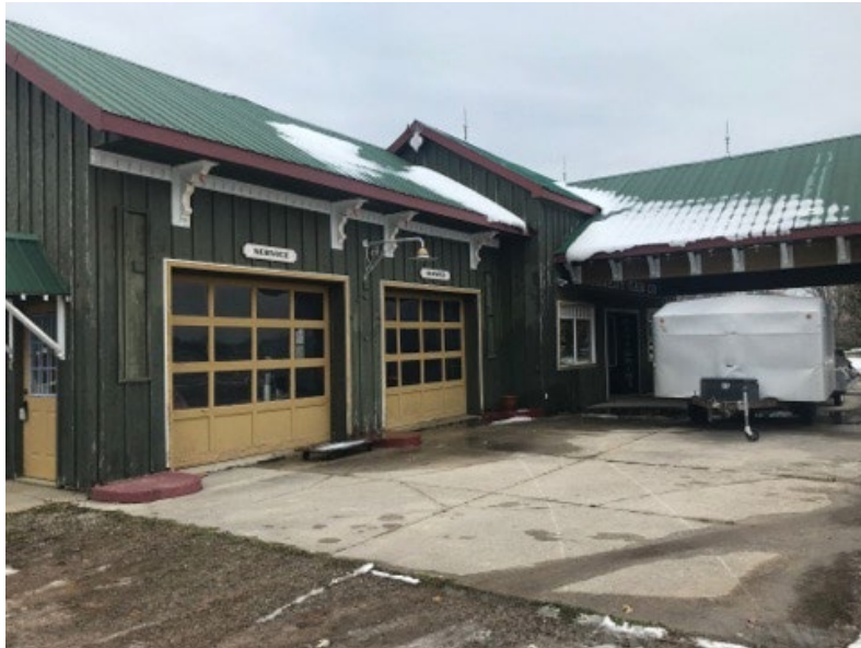
Photo 7– View of Building B, facing northeast. Note: service garages.
