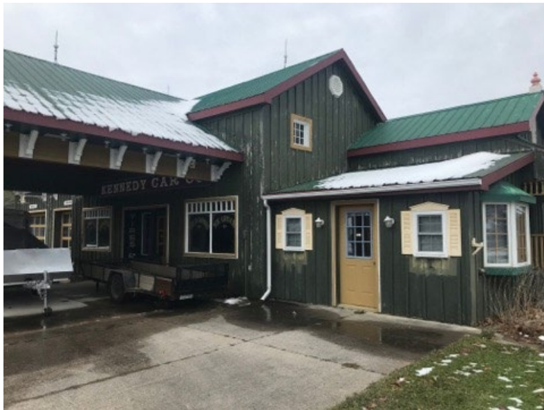
Photo 8 – View of Building B, facing northwest.
