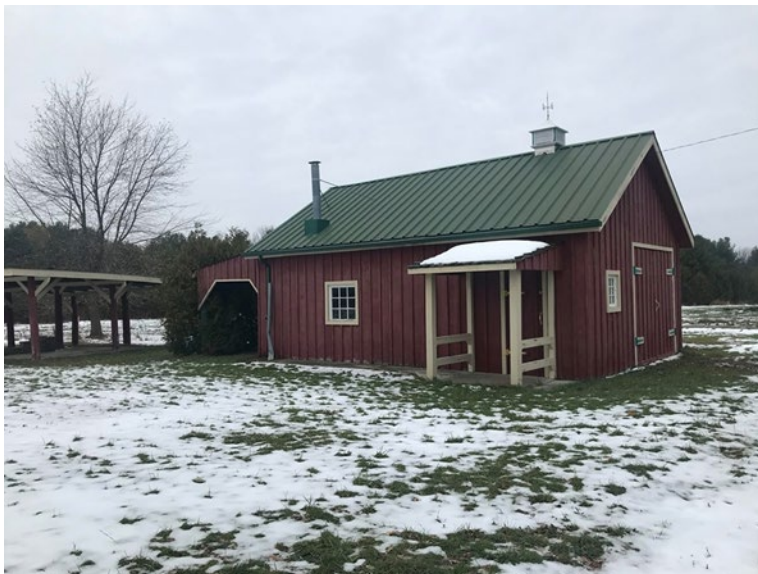
Photo 18 – View of Building E used for storage, facing northwest
