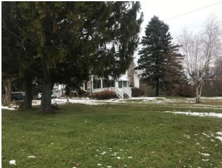
Photo 6 – View of Building A, facing northeast.
