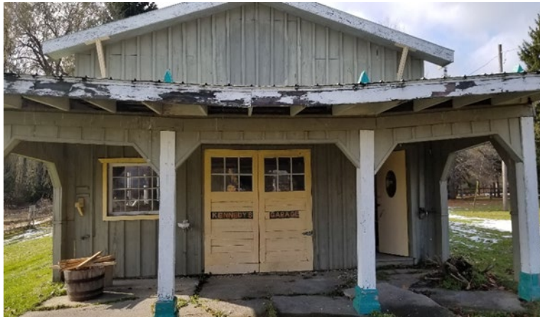
Photo 14 – View of Building C used for storage, facing west. Note: suspected former vehicle maintenance/service garage
