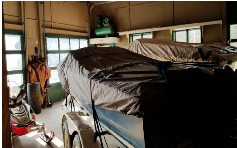
Photo 10 – View of the garage portion of Building B utilized for storage.
