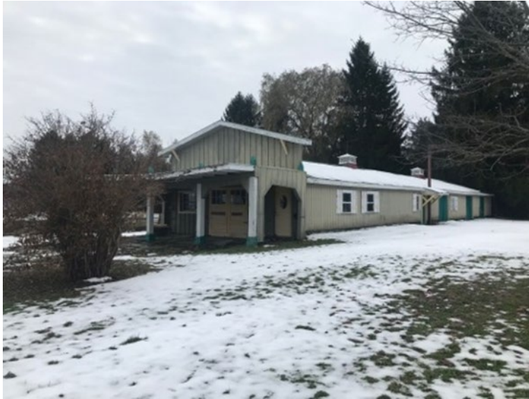
Photo 13– View of Building C used for storage, facing southwest
