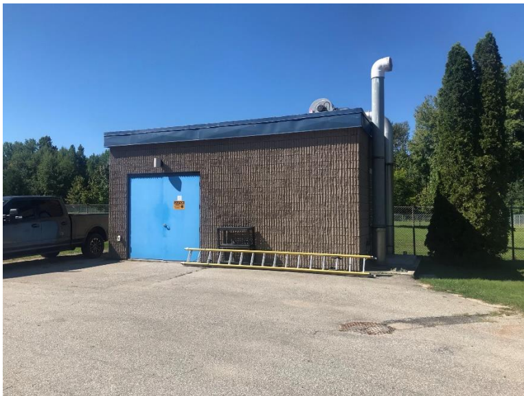
Figure 10: Sewage pumping station, looking west (A.S.I. 2022)
