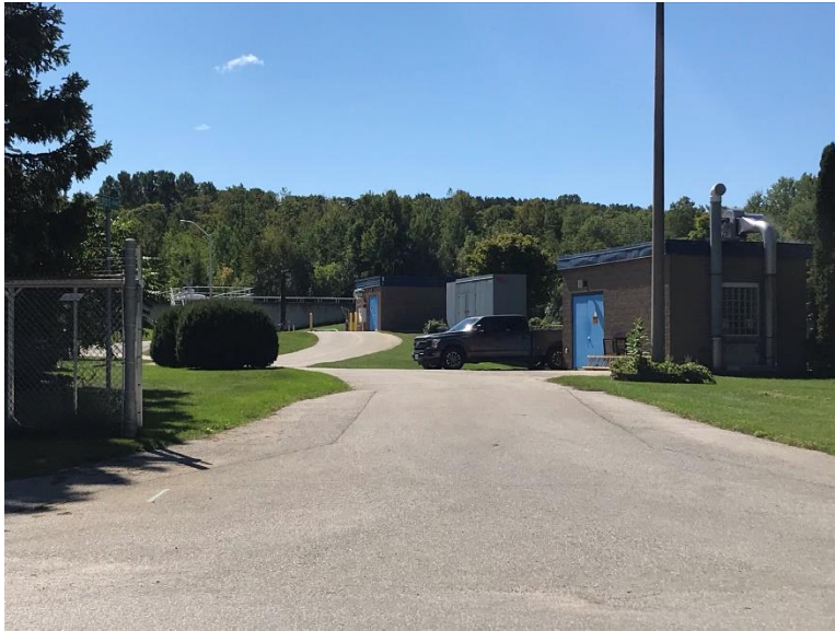
Figure 9: Entrance drive to the subject property, looking south (A.S.I. 2022)
