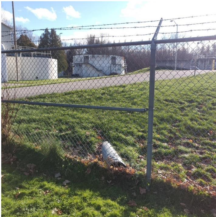
Image 7: Wastewater Treatment Plant drainage and facility components, disturbed, no potential.
