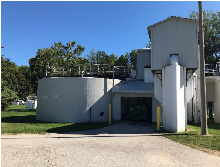
Figure 14: West elevation of aeration tank with inlet pipe at right (A.S.I. 2022)
