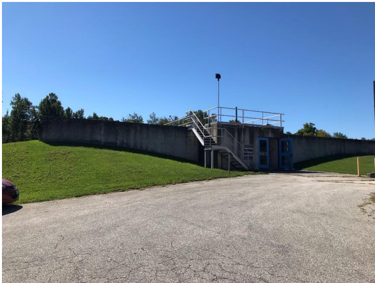
Figure 18: North elevation of the biosolids storage and treatment facility (A.S.I. 2022)
