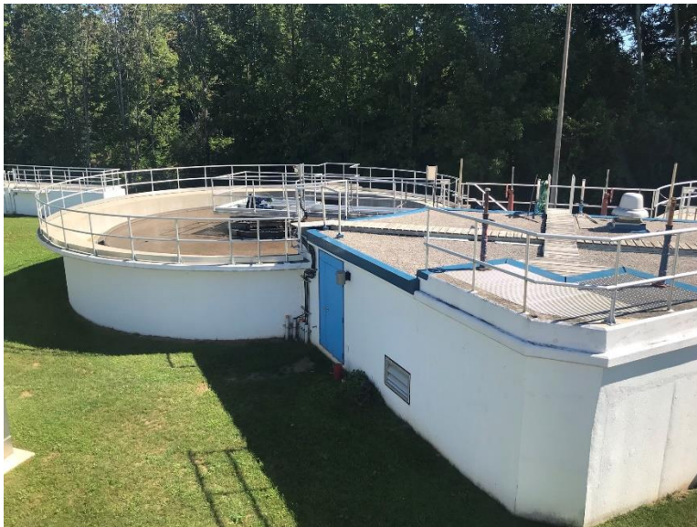
Figure 16: Secondary clarifier, looking east (A.S.I. 2022)
