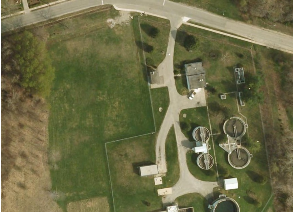
Image 14: 2010 aerial imagery showing grassed field to the west of the Wastewater Treatment Plant.
