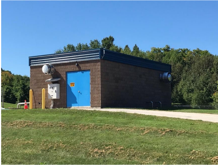
Figure 21: Blower building (A.S.I. 2022)
