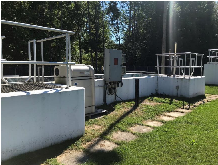
Figure 20: Ultraviolet disinfection channel (A.S.I. 2022)
