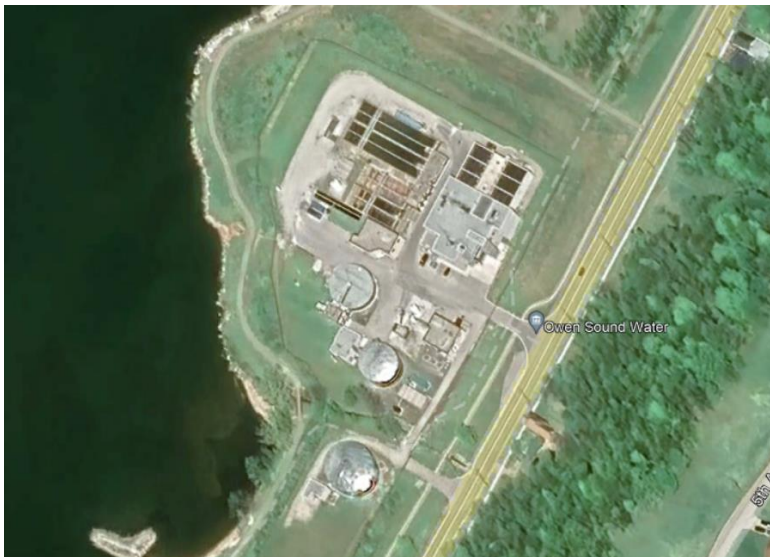
Figure 28: Satellite imagery of the Owen Sound Waste Water Treatment Plant (Google Maps)
