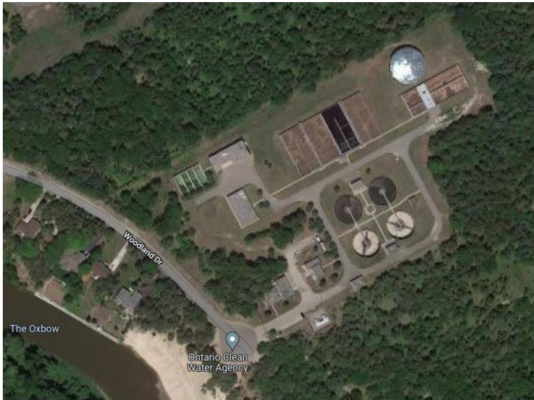
Figure 30: Satellite imagery of the Wasaga Beach Water Pollution Control Plant (Google Maps)
