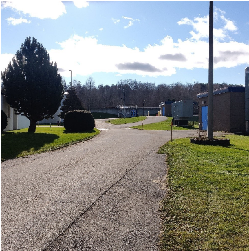
Image 2: Wastewater Treatment Plant, disturbed, no potential.
