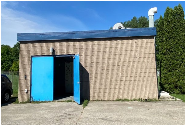
Figure 3 – Raw Sewage Pumping Station
