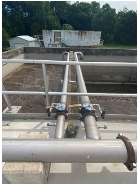
Figure 8 – Aerated Digester
