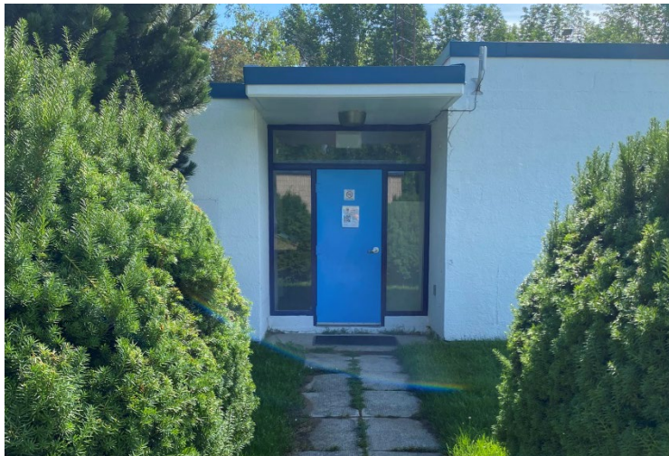
Figure 2 – WWTP Administration Building
