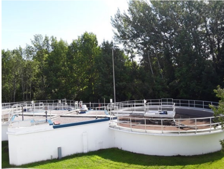
Figure 6 – Secondary Clarifier
