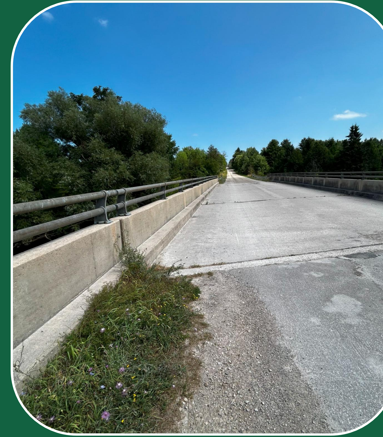
View of Structure Facing East
