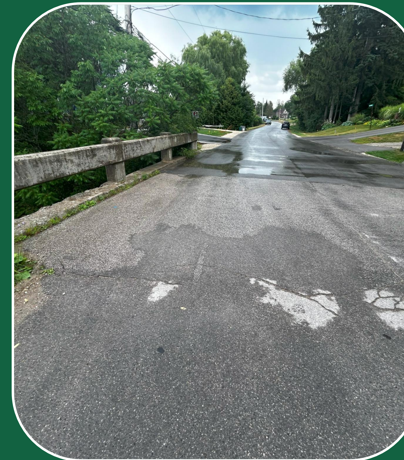
View of Roadway Facing South
